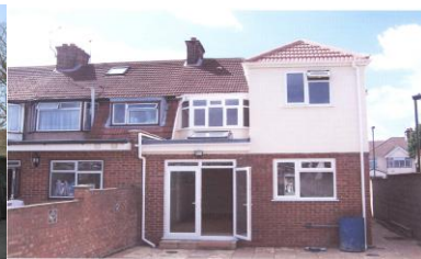
2 Storey rear extension Burns Avenue, Southall
