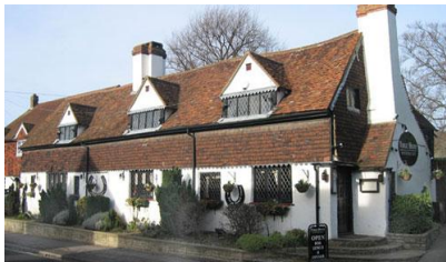
Rear extension & internal alterations The Forge House Restaurant, Kent.
